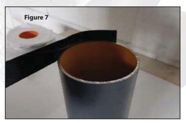
7.5 Draw the epoxy tape around the pipe with slight and uniform tension, to a slight overlapping. If there is a gap, loosen both sides separately and draw the tape with higher tension until it overlaps (See Figure 8).
